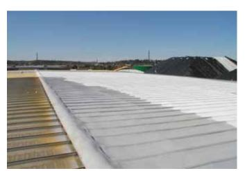
After an acid-etch surface prep, the crew used 1/2" nap rollers to apply a primer coat of Roof-Tek 7500 Acrylic Primer. Then, using a Graco/Gusmer H-20/35 Pro and 2 Gusmer H-2s fitted with GX-7 guns, they spray-applied a 1 1/2" layer of BASF-FE Roof-Tek RT 2716 Series, 2.7 Roof Foam. This was followed by an acrylic latex elastomeric topcoating of Tek 4200, applied at 27 to 30 mils DFT, with Graco 733 airless sprayers.
