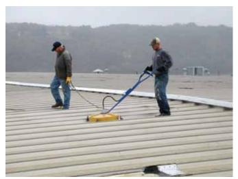
Arriving on site, the Kohls crew discovered a large corrugated metal roof — approximately 127,000 sq. ft. — covered in a variety of failing coatings. In addition to 49 leaking fiberglass skylights, 108,000 sq. ft. of the roof was covered in fully adhered EPDM membrane, while the remaining 19,200 sq. ft. was covered in gravel built-up.
